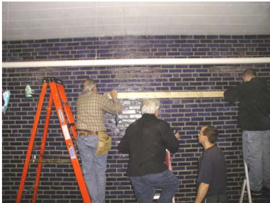
__Installing Cabinets at the Y – January 2007
